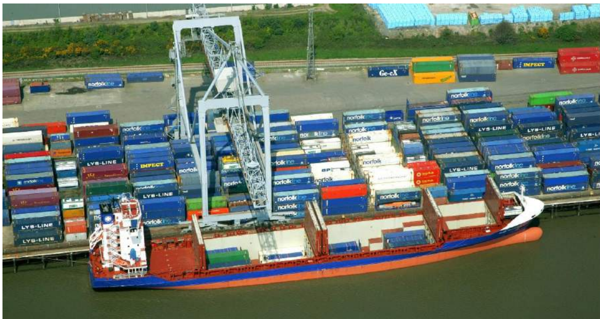
Figure 2 Containerised cargo is discharged/loaded by using 2 high speed wide-span gantry cranes
