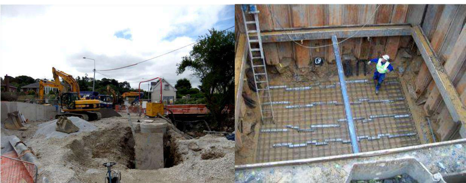
Works to a pump chamber in Mallow
